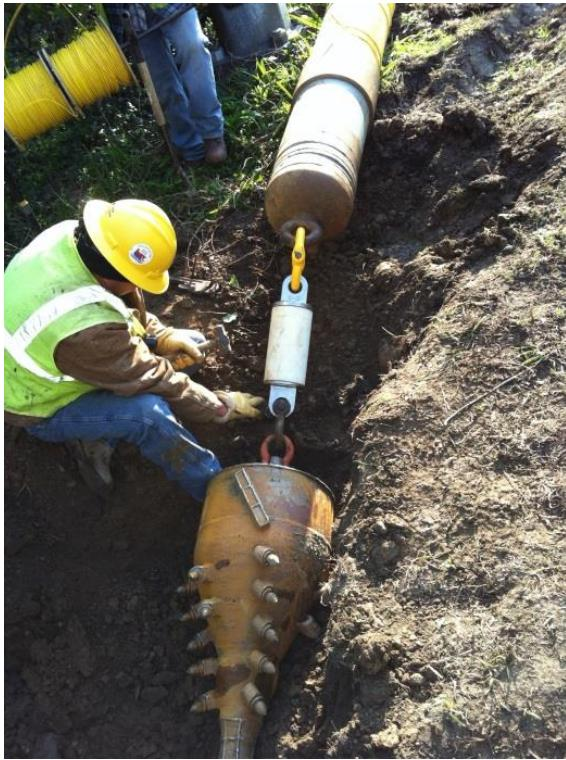
The DigiTrak® F5® TensiTrak® Pullback and Pressure Monitoring System provides critical installation data to HDD operators, allowing real-time monitoring of product pull force and downhole mud pressure without a wire. Real-time pull force/tension monitoring helps prevent damage to the product and costly reinstallation. Knowing downhole mud pressure assists in preventing inadvertent fluid returns or, even worse, road buckling.
