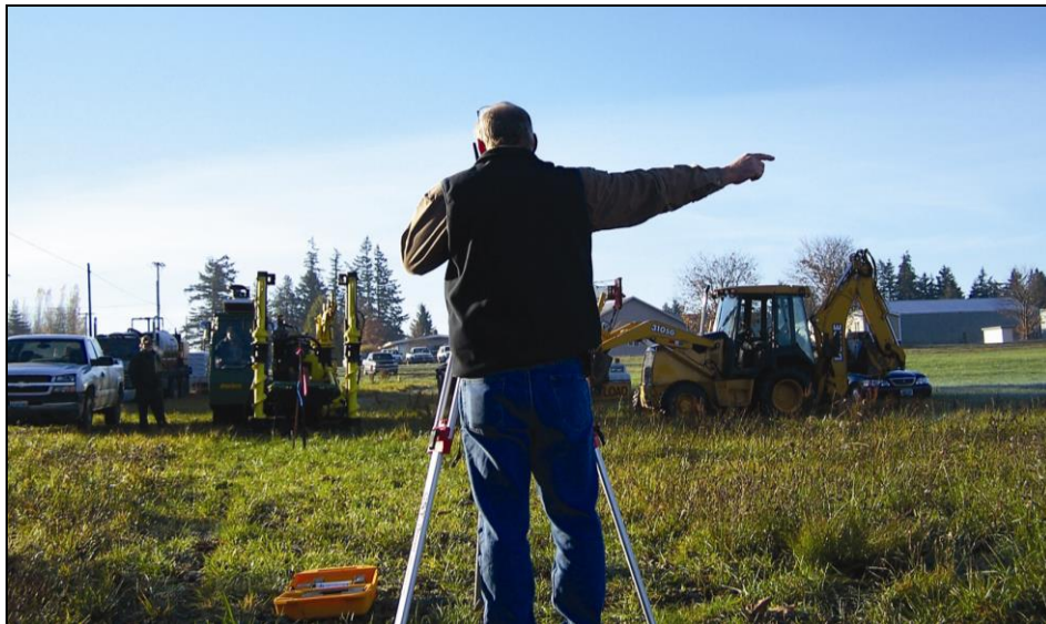
Aligning Drill to Marked Bore Path
