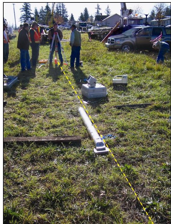
Aligning Drill to Marked Bore Path
